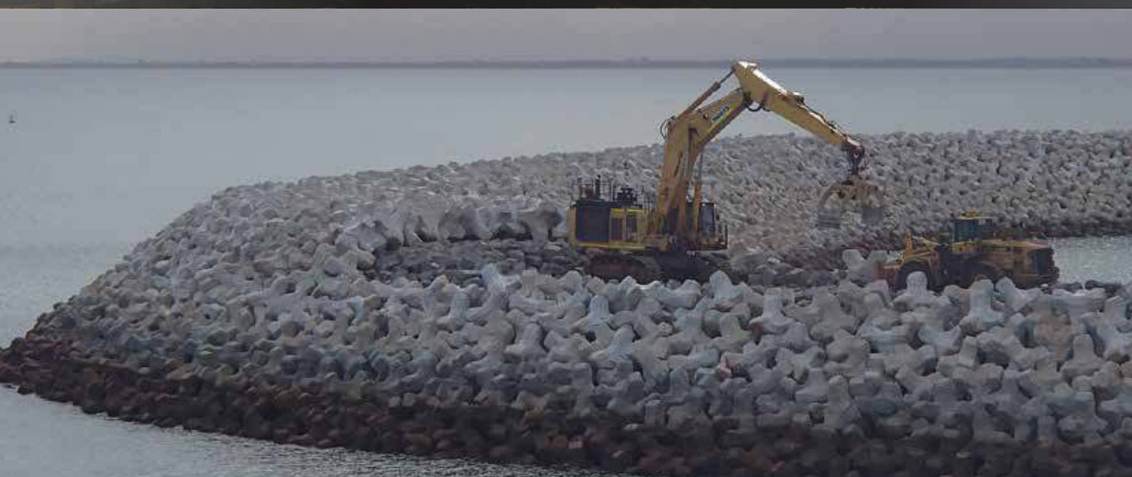
Special application Breakwater block Grapple used on 125 tonne Excavators Picture of Onslow West Australia , Wheatstone Project LNG Plant
